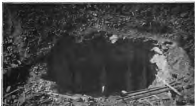
C. NO. 2 SHAFT IN LAKE LODGE. SHOWS THREE COMPARTMENTS.
